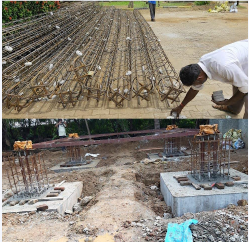
Foundation setup for weather radar installation
