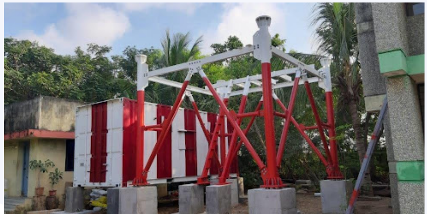
Weather radar foundation construction in progress
